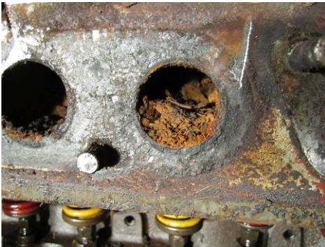
Exhaust port with manifold removed. This could have been a mess on start up.
