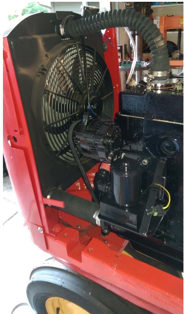
Painted water pump and alternator installed
